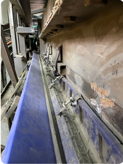
Installation of AirScrape together with SureSupport. This combination improves material absorption and ensures optimum tightness.
